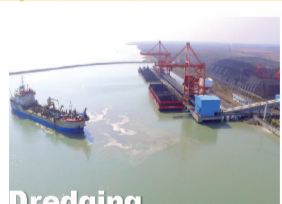
Dredging Coal-powered power station port facility dredging PT Huayuan is a power plant with a capacity of 3000 MW using low rank coal/low-rank coal as steam which can then drive turbines and produce mechanical energy for the generator process into electrical energy.
